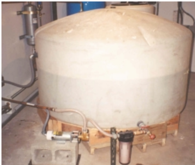
500-gallon water storage tank
