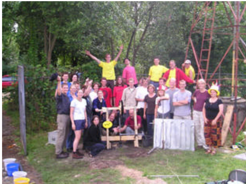
The participants of the T-Week pose at their newly constructed well, rope pump and solar collector.
