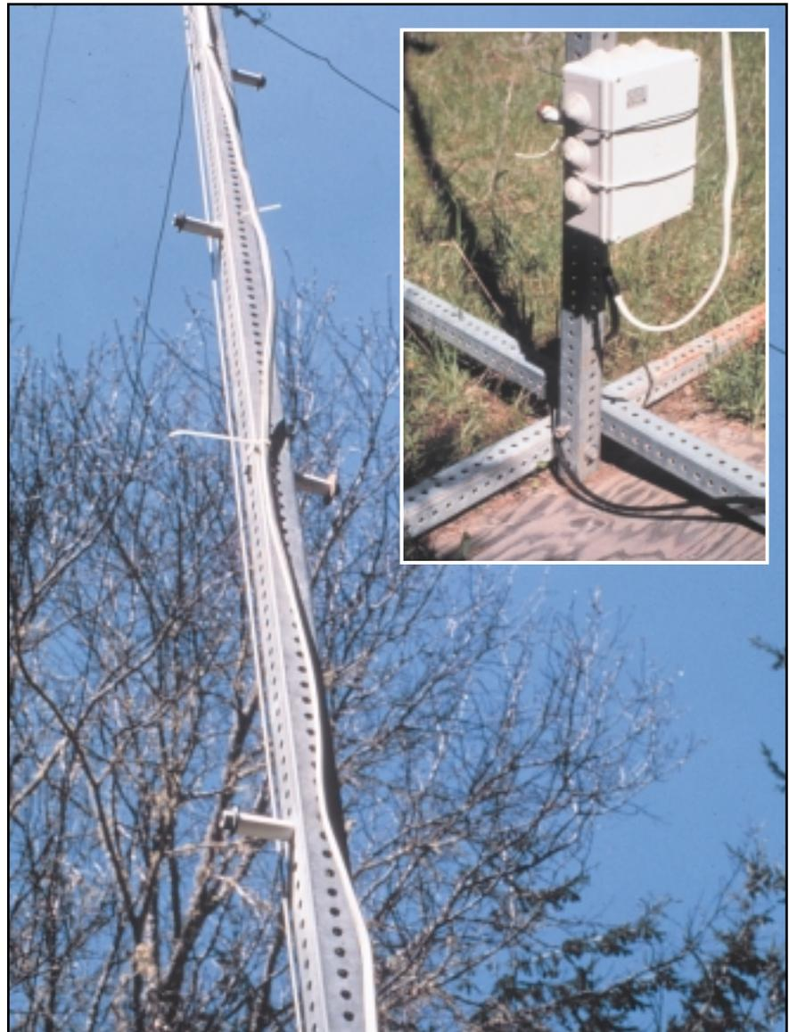
Above: Foot pegs facilitate tower climbing. UV-rated electrical cable is cable-tied to the tower. Inset: An LCB mounted at the tower's base assists the pump in early morning startup or in winter sun.
