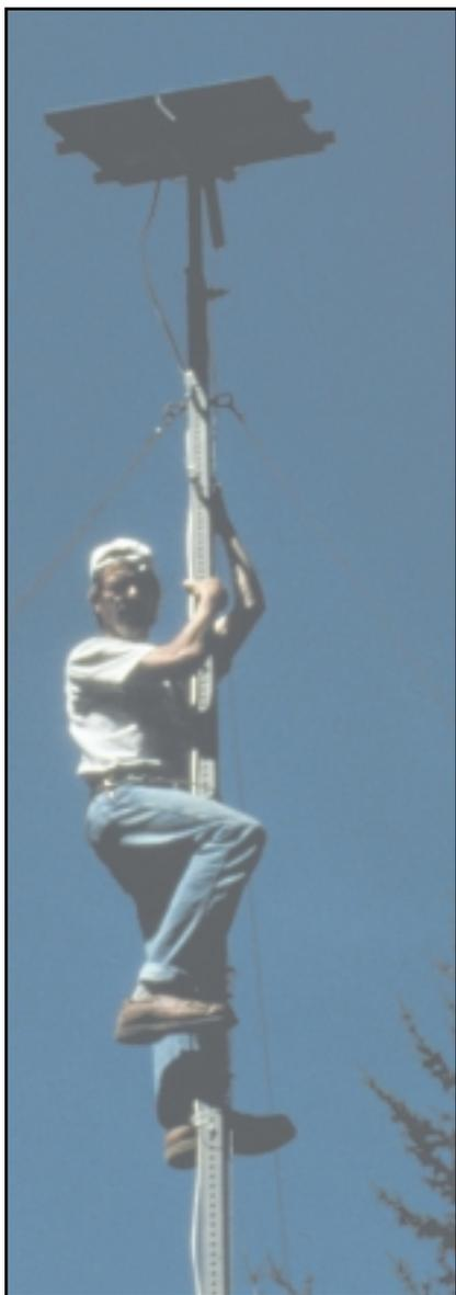
**Above:** The 42-foot tall tower is slender but is easily climbed to clean the modules and inspect the hardware and wires. (Always wear a tower belt!)
