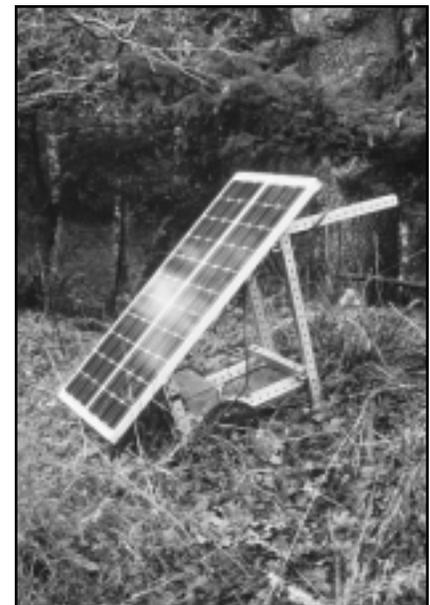
The original installation—two modules on a homemade cart to power a pump in the spring tank.
