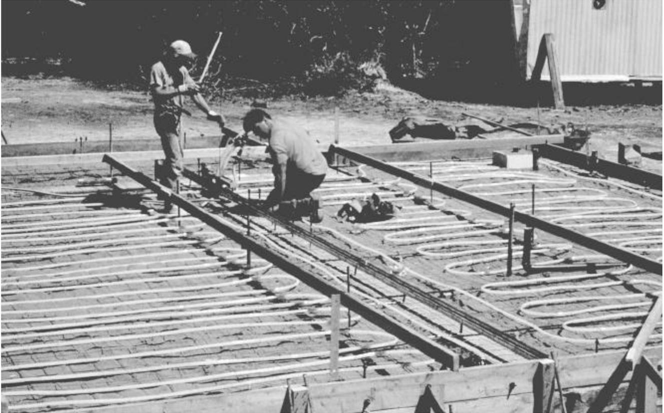
The McMillan foundation is inlaid with insulation and tubing and checked for leaks prior to pouring the slab.
