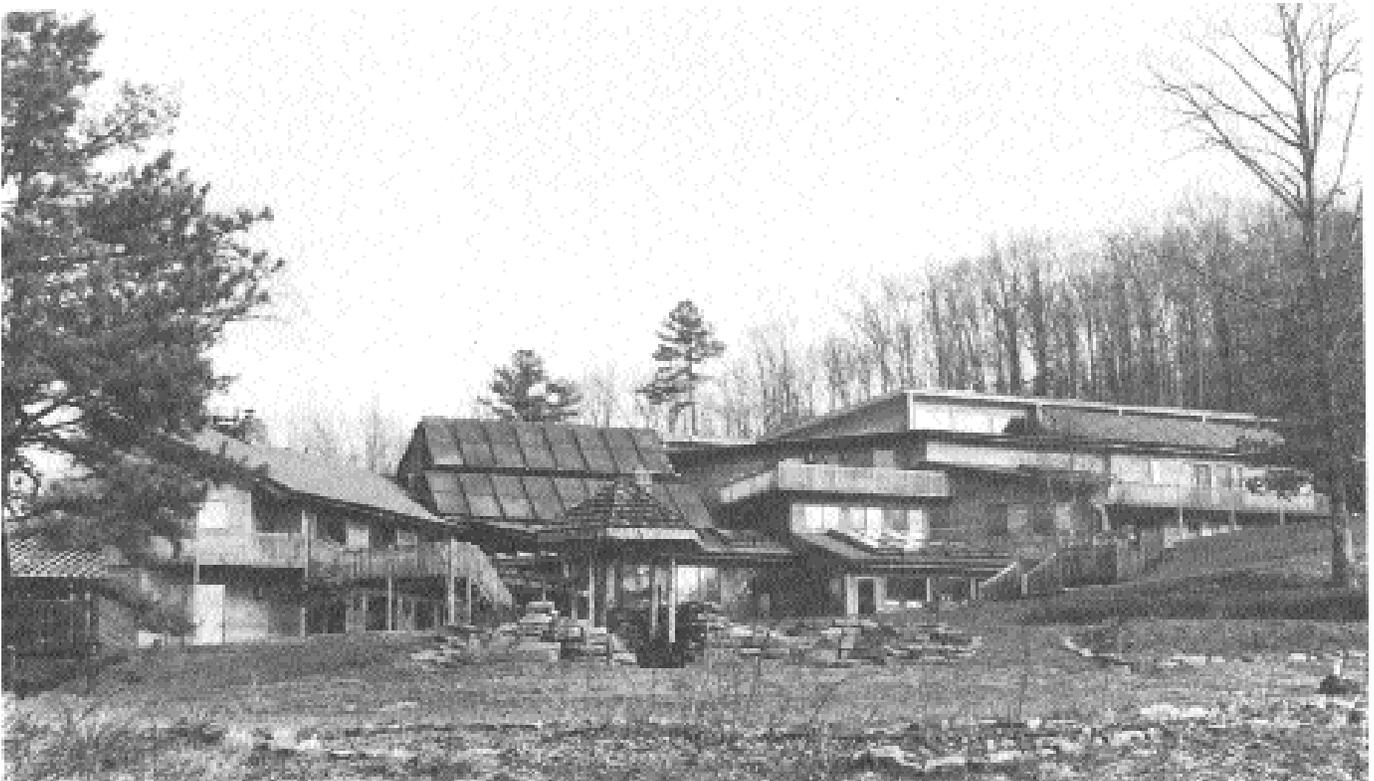
*The energy-efficient education center at Meadowcreek nestles into a hillside. Solar hot water collectors are left-center. Fixed 5KW photovoltaic array is at right.*
