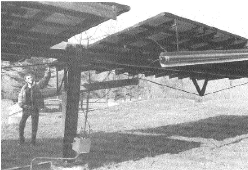
*Meadowcreek's director, Luke Elliott, explains how a freon-powered tracking system works on the ground-mounted 5KW photovoltaic array. The gas in light-fixture-like tubes at front and at the rear of panel expands in the sun warmth to push at a piston in the container visible center-photo.*
