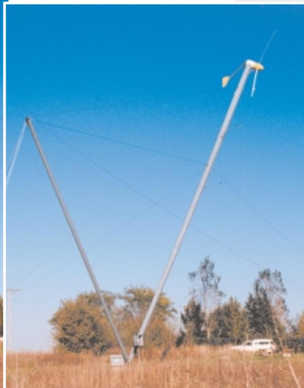
wall. For large windplants or taller towers, I use 5-inch schedule 40 pipe, which is well casing. We encourage the customer to buy either type of pipe locally to save on shipping costs. The kits vary from basic to complete. Most include the pipe couplers, guy wires, attachments, turnbuckles, pulleys, and other rigging.
