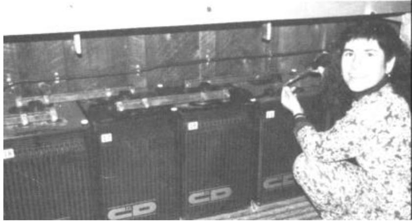
*The author using a hydrometer to test the charge on the used telephone company batteries in which the electricity is stored. Each battery weighs 400 pounds.*
