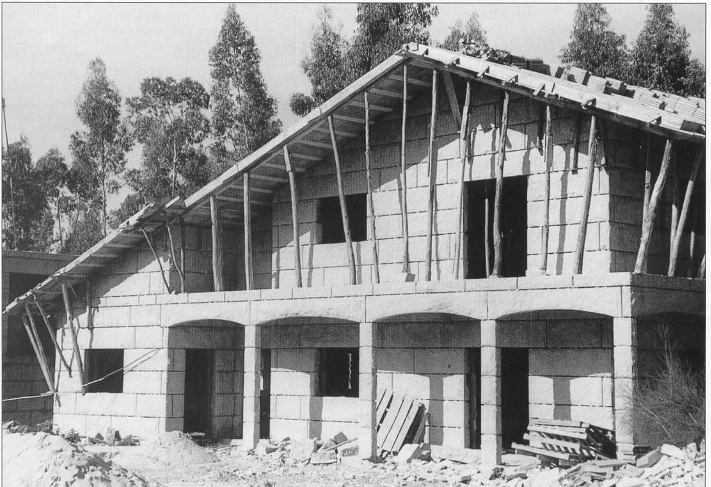
Figure 8: House in Alpendurada near Oporto, Portugal
