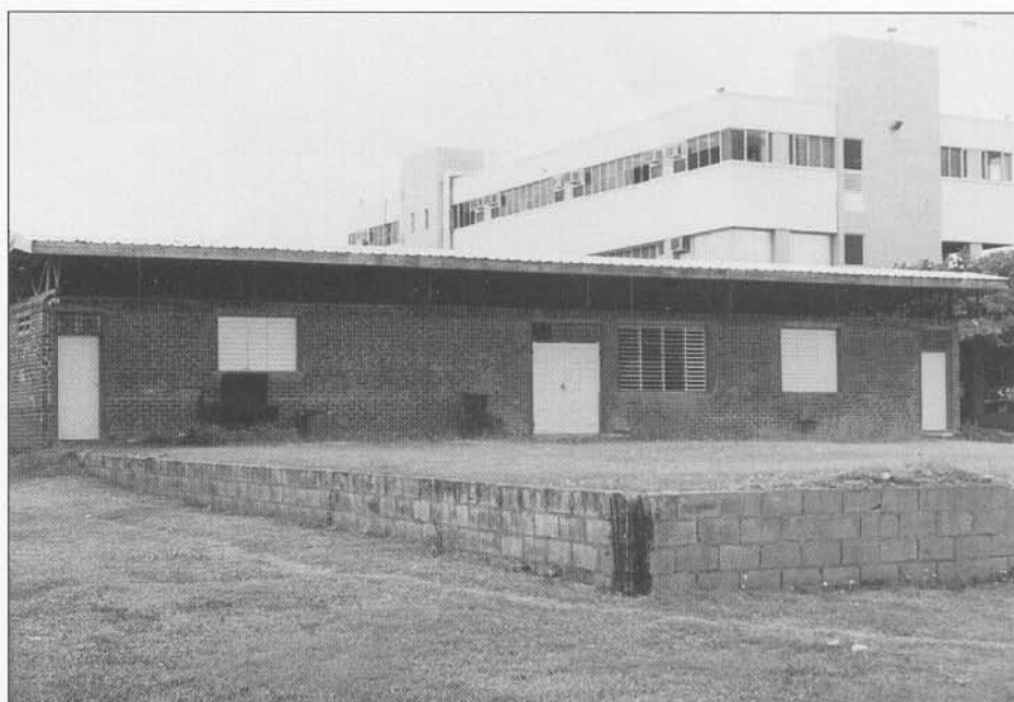
Fig. 2: Front view of the "Red Mud" demonstration building at the Jamaica Bauxite Institute (Sports Pavilion)
